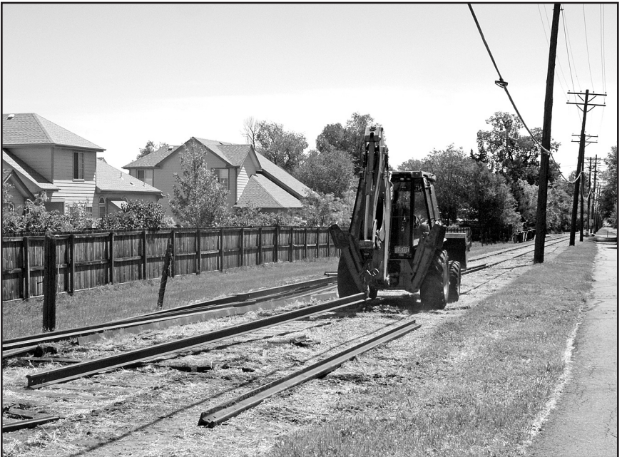
Removal of the Associated Railroad line to Lakewood began on the west end. Here we see rails being removed and loaded just east of Kipling Street. – Two photos © 2007 Darrell Arndt.
