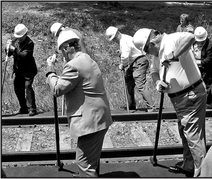
Dignitaries with spike pullers remove spikes from the Remington Arms Spur off the former Denver and Intermountain line. – Photo © 2007 Bob Wilson.
